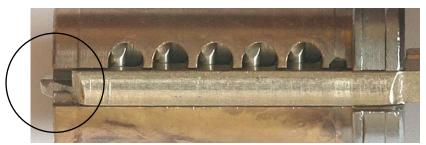
**Details of the bottom of the Twin V10 keyway with the key inserted** Note: The specific tip of the key in this system.
